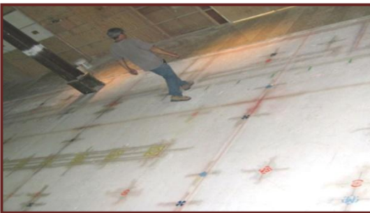
Painted lay out for all the trades
